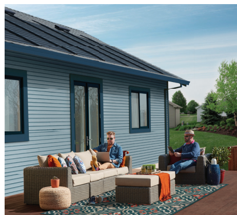
Experienced GAF-certified contractors handle the work on the roof.
